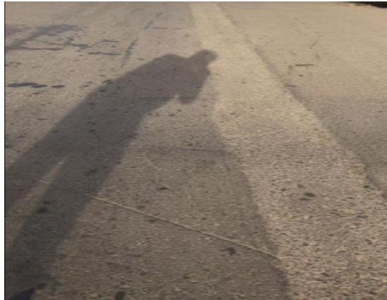
Figure 7. Patching (Location No.4).
